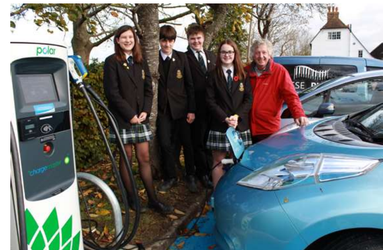
BELOW Rapid Charger installed at Kings Academy, Ringmer
